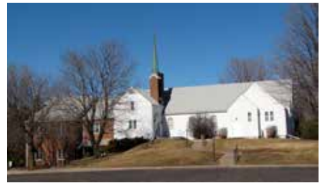
Maplewood Covenant Church Maplewood, MN / 1932-2015
